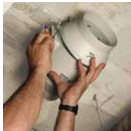
Place the impeller and motor assembly.
