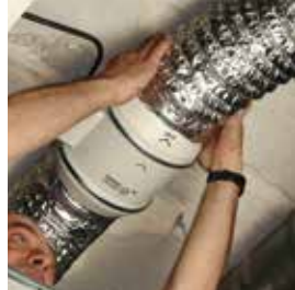
Connect the ducts.
