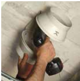
Fix the support bracket.
